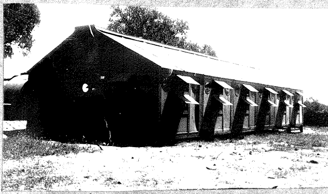
Operations & S-2 Bldg.
